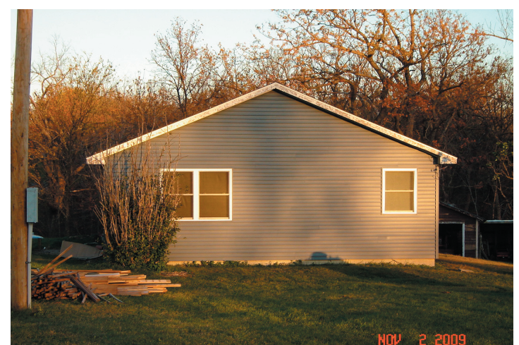
The house - new roof, windows and vinyl siding.
